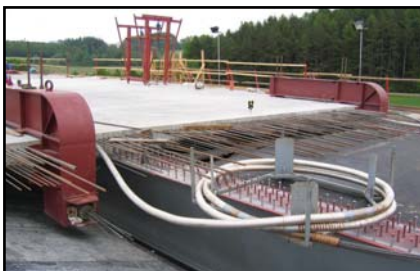
▲ Pulling tendon brackets.
