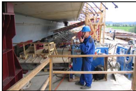
▲ Pulling tendon, launching control desk.
