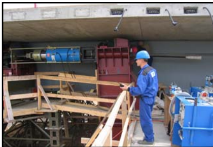
▲ Smooth slab forehead after grouting.
