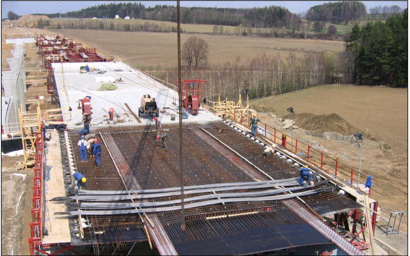
▲ SO 6-4 Tendon Preassembly.
