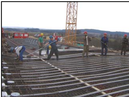
▲ SO 6-4 tendon placing.
