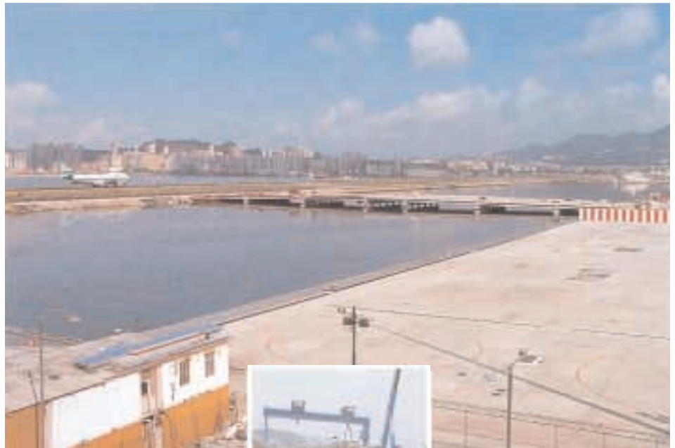
Precast T-beams proved to be the most cost-effective solution for this bridge
