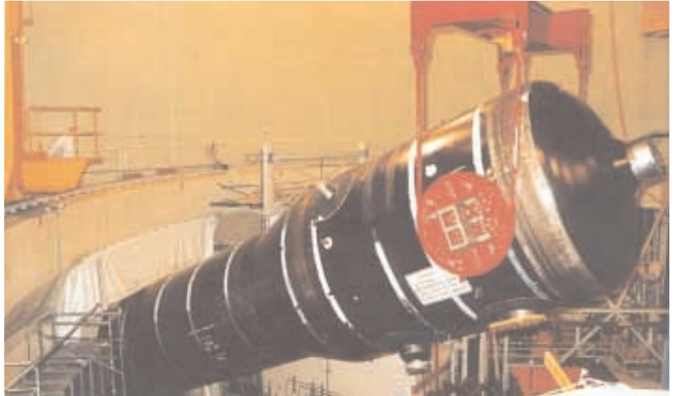
Exchange of steam generator
