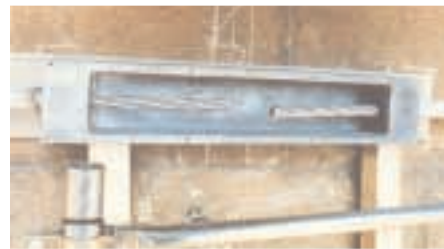
Circumferential prestressing single strand anchorage body
