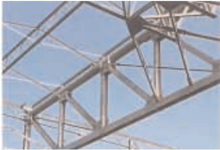
Bottom tension chords reflected up for stressing
