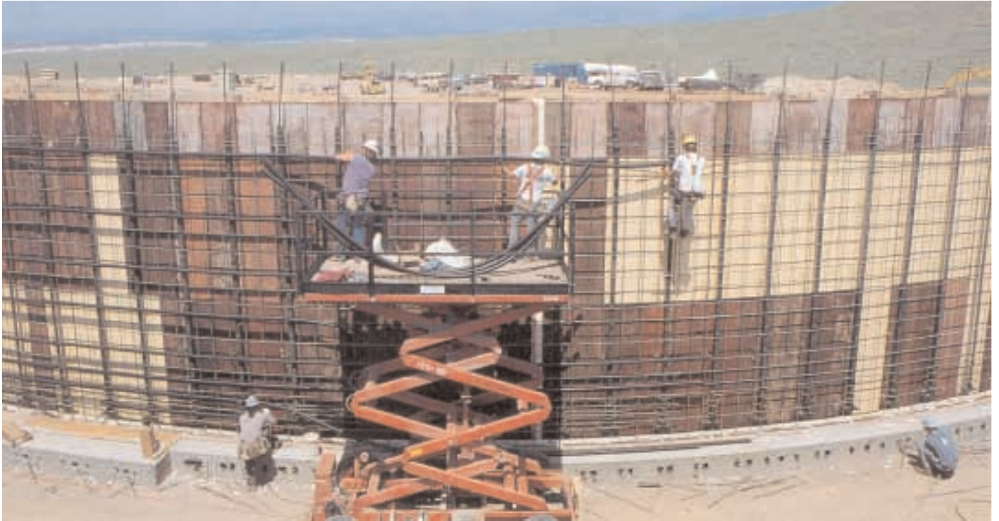
Front view of the Denver Tank
