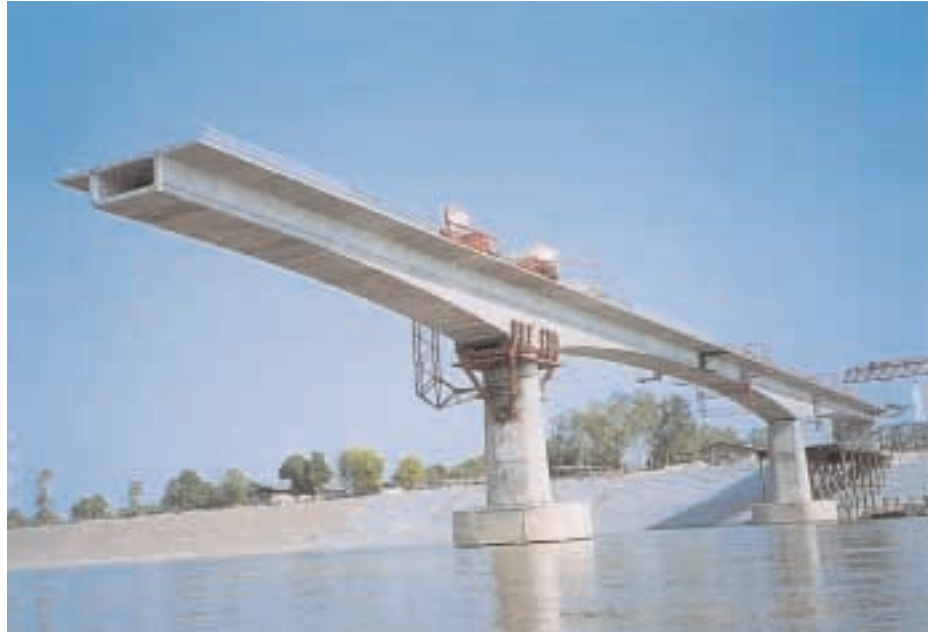
Balanced cantilever construction at Mekong River Bridge
