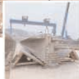
Precast T-beams proved to be the most cost-effective solution for this bridge
