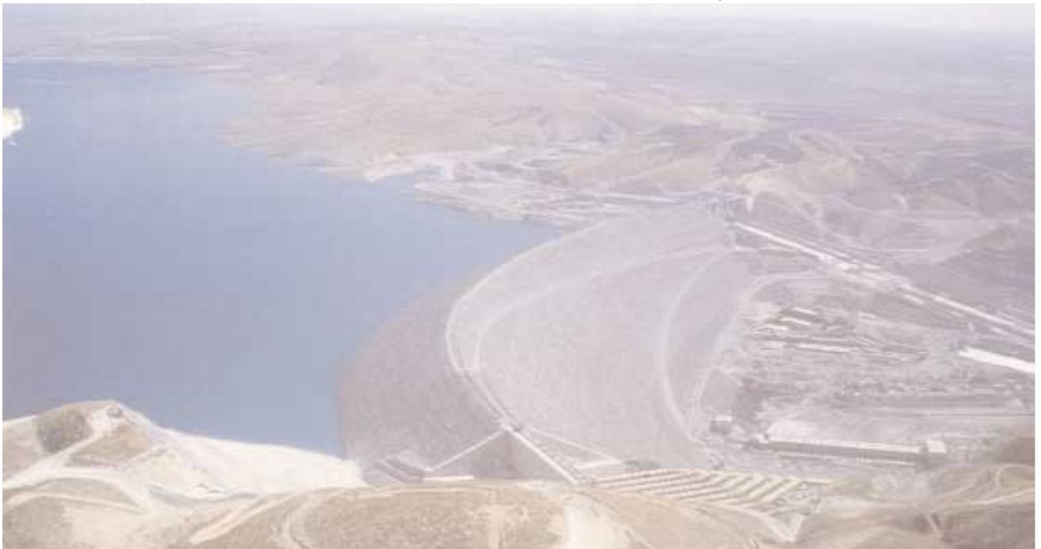
Atatürk Dam has an embankment volume in excess of 84 million cubic meters.
