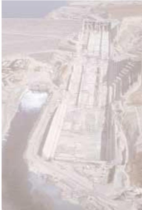
Spillway and stilling basin. sion protection of the free length of a considerable number of anchors. A packer that permitted pressure grouting of the anchors was specially developed to overcome this problem. █
