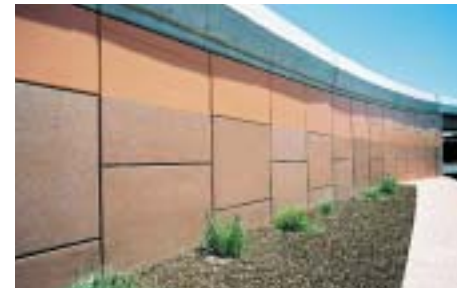
Nundah Bypass, Queensland, Australia.
