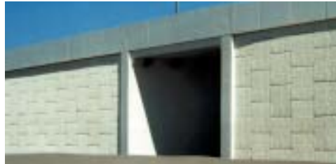
Truck Road, Contract No.2, Dubai.
