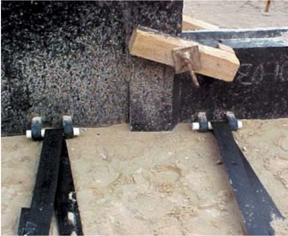
Friction tie installation.
