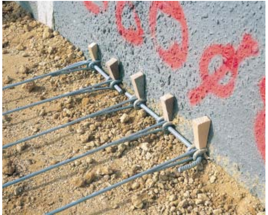
Simple moment free pinned connection to panel clevis loops.
