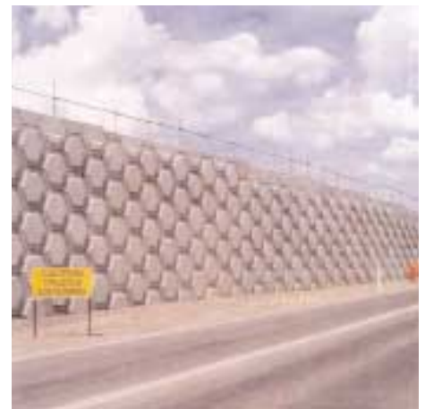
The VSL Retained Earth System - an attractive and economical solution for difficult embankment and retaining wall problems.
