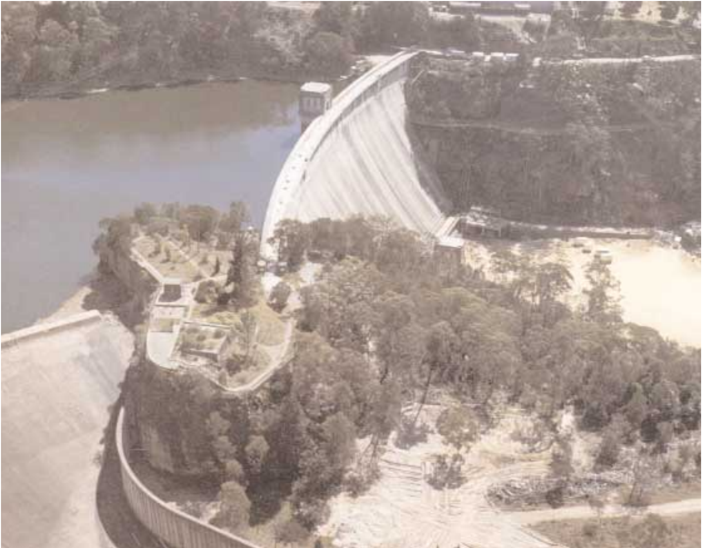
Nepean Dam safety improved by the world's largest and longest permanent ground anchor.
