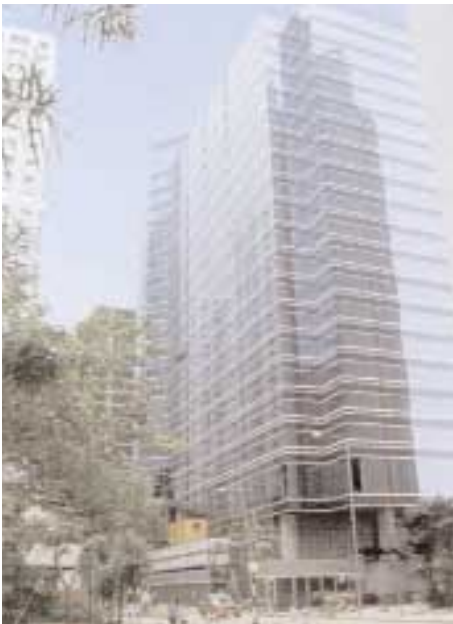
City Plaza, "CP4" after completion
