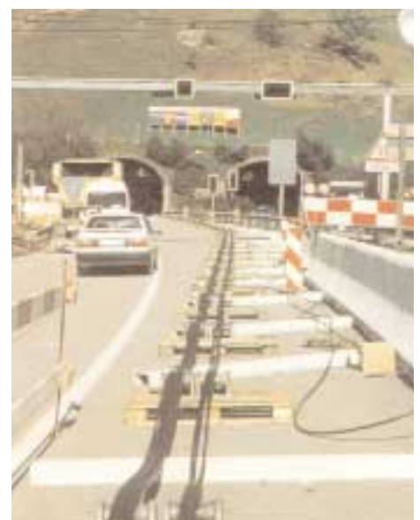
VSL's monostrand concept for external tendons provides the strands with corrosion protection during fabrication and permits extremely long tendons.
