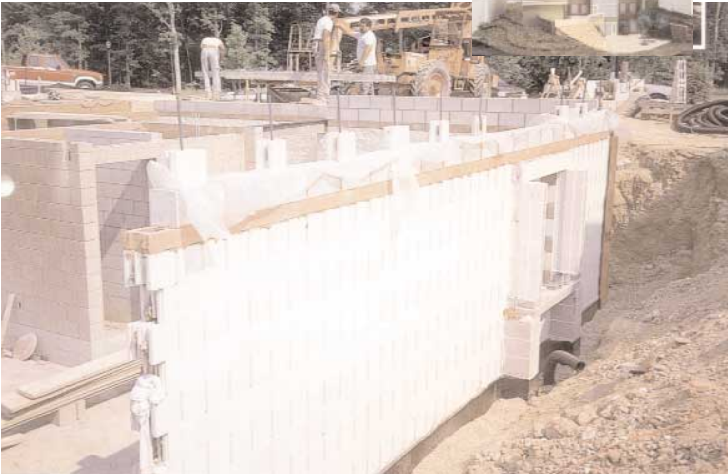
Vertical post-tensioning strengthens masonry walls and furnishes resistance to imposed deformations from lateral earth pressure.
