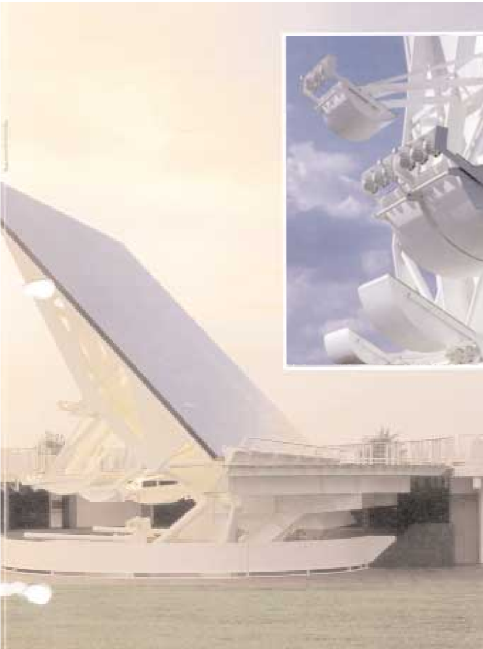
Mirrors attached to steel trusses at the rear of the rotating wall track the sun and reflect its light through the cut out names in the wall's granite.
