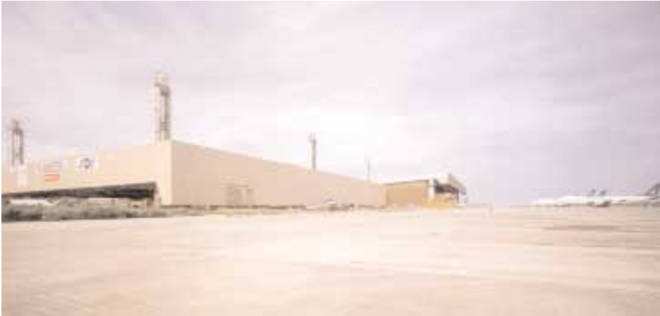
The 3,000 tonnes roof structure was lifted into position with a levelling accuracy during lifting of 2 mm.
