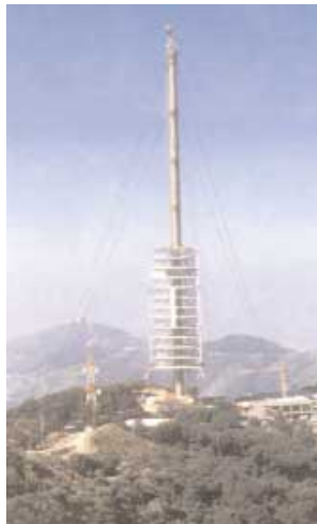
12 storey service building assembled on ground, shown being lifted 85 meters to its final position.
