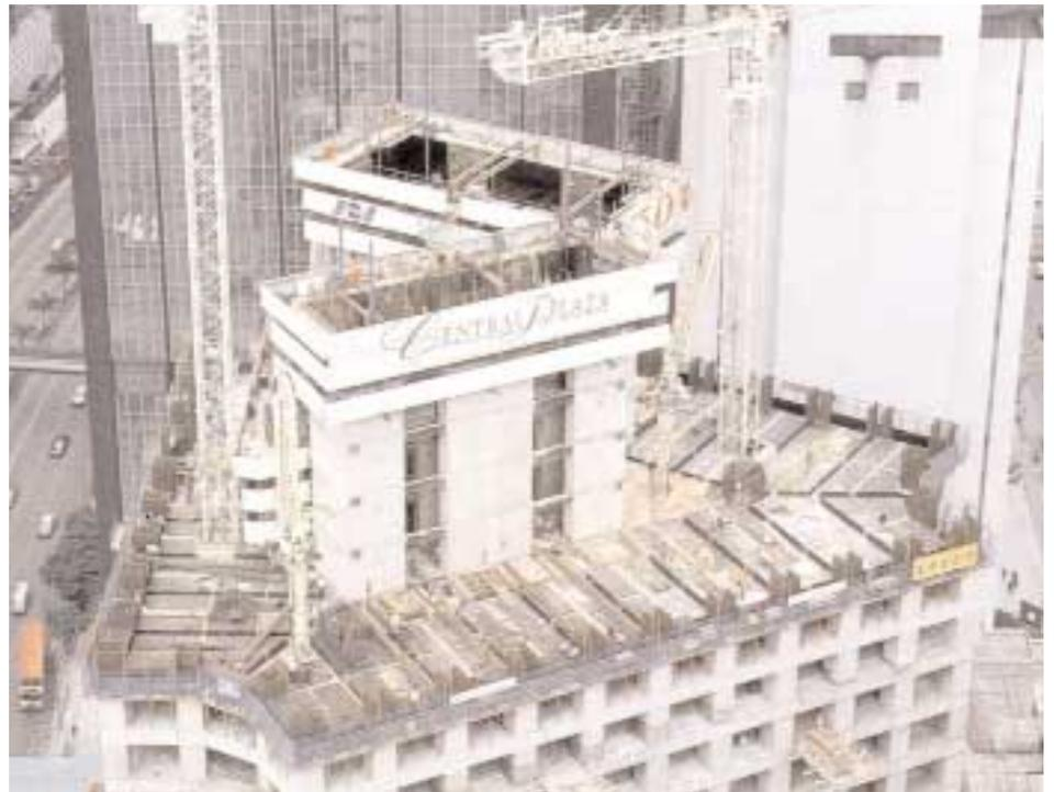
completion in February 1992, only 26 months after inception. For the largest tower the climbform features single storey height forms covering 654 square metres of core wall surface and incorporates 117 tonnes of reinforcement steel with a concrete pour of 306 cubic metres.
