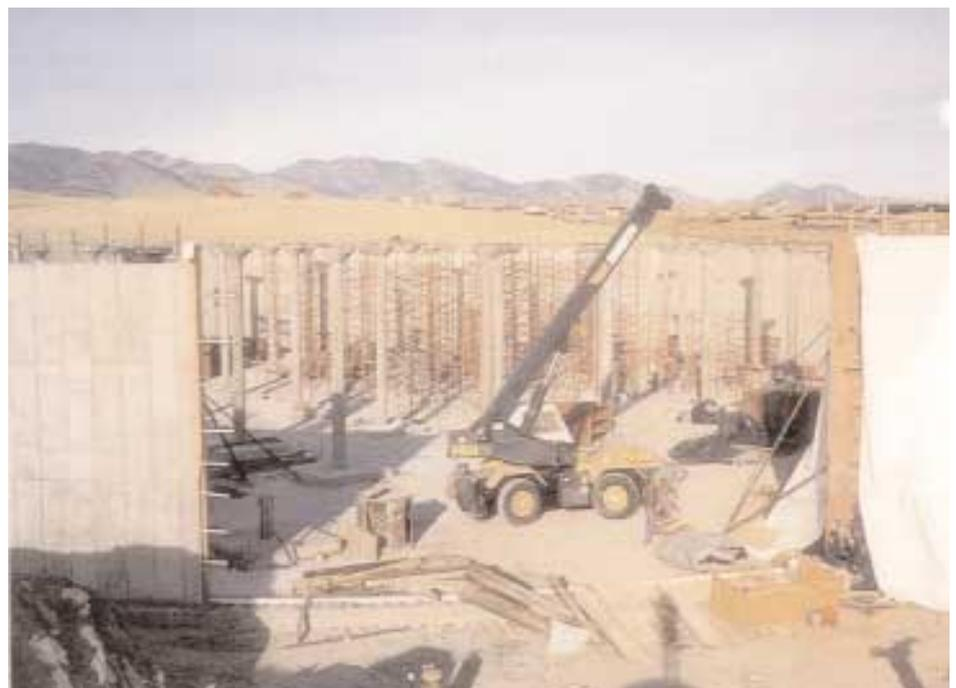
Colorado tank has post-tensioned floor, wall and roof.
