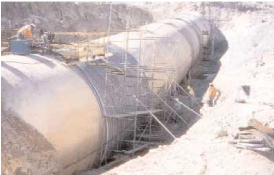
**Corroded prestressing wire was replaced by corrosion-protected VSL monostrands. The monostrands are epoxy coated, grease coated and encased in high-density polyethylene sheaths.**
