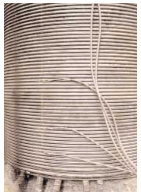
Wire wrapped column base after testing.
