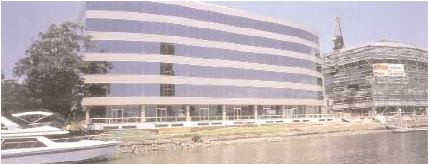
Post-tensioned structural system allowed 2.7 m high ceilings and 1200 m 2 of column-free space on each floor.
