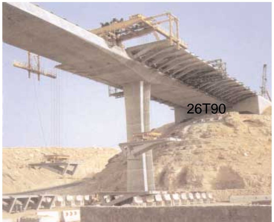
Lifting operation for precast side frames.
