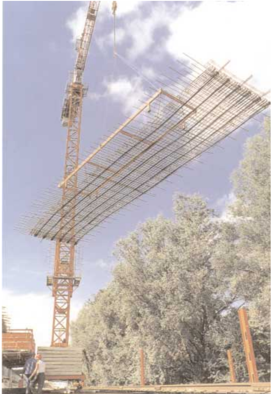
Site prefabricated reinforcement, including strand and anchorages, speeded composite deck construction.
