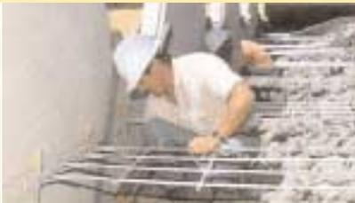
4 • Connecting the mesh with the loop clevis thanks to a dowel bar
