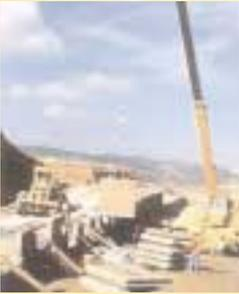
2 • Placing the panels using a standard crane
