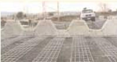
4 • Placing the reinforcing mesh
