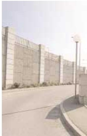
Each wall segment is a single panel with a partial raised relief and sandblasted finish that perfectly follows the line of the road profile. The works started in November 1998 and will be completed in Spring 1999. ■
