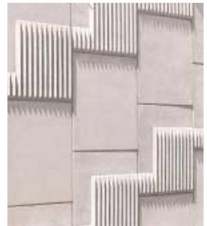
The Cayuga Street walls were supplied to the conforming architectural requirements of a 1.5-m x 1.5-m panel with a stepped rib pattern finish and represented nearly 70% of the total area of wall. All remaining walls were supplied in a smooth hexagonal finish. The total wall area was over 3,000 m<sup>2</sup> with a maximum wall height of 6.5 m. ■
