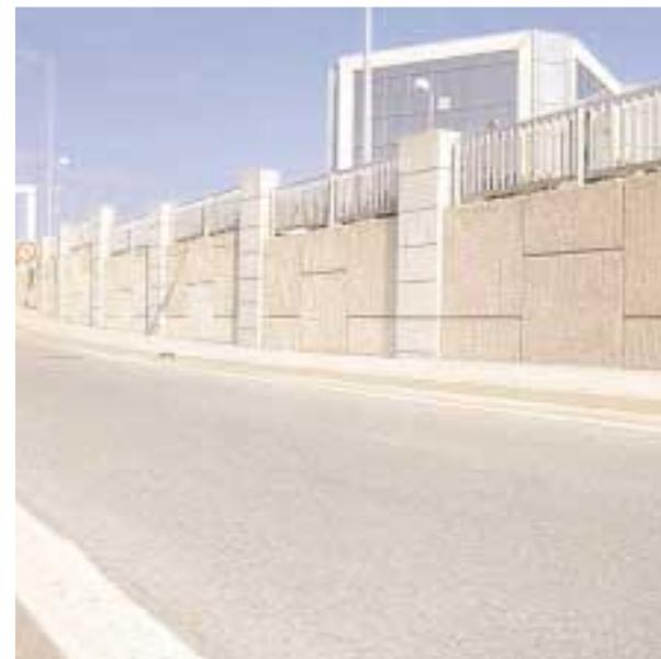
These walls, topping at 6 m for a surface area of 1,800 m<sup>2</sup>, were designed so that their facings exactly matched the pattern chosen by the architect. No less than 80 different types of precast concrete panels were required to satisfy this demand.
