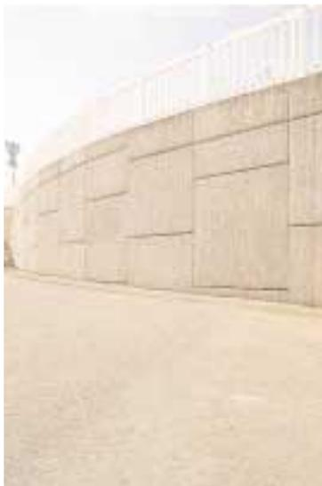
embankment, allowed for a 15% cost reduction for the backfill when compared with competing reinforced soil systems.
