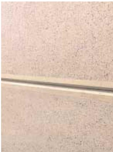
VSL was awarded the contact to design and supply the Retained Earth Walls based on a 2-m x 1-m panel module with in-line horizontal and vertical joints. The conforming arrangement presented difficulties for wall installation. Therefore, VSL's successful alternative using a 2-m x 2-m panel with a false joint provided a workable solution and consistency with the architectural requirements.
