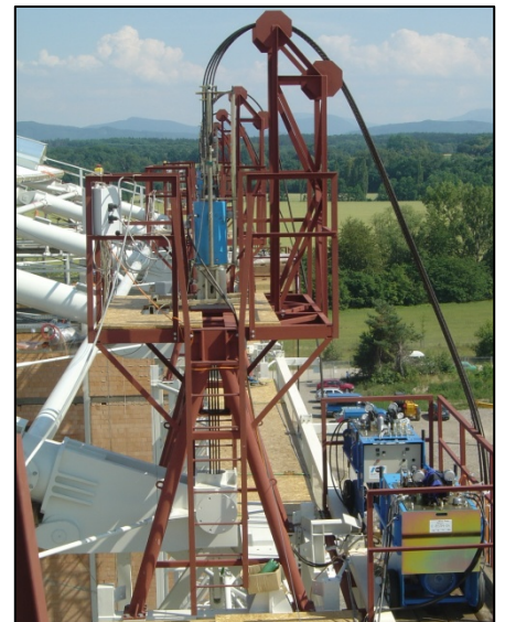
▲ The columns were fitted with VSL SLU 120/500 lifting units.
