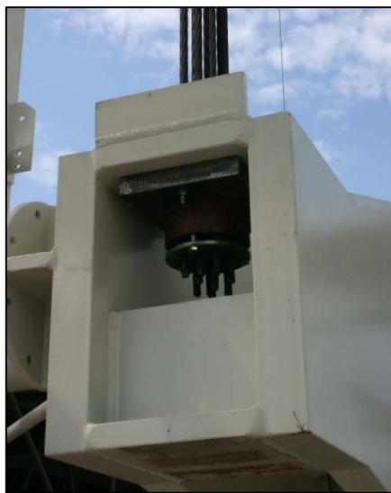
▲ Anchoring the cables using anchor heads
