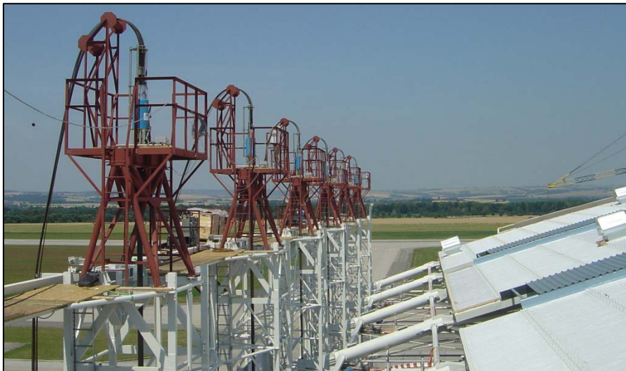
▼ SLU 120/500 hydraulic lifting units carried out the lift.
