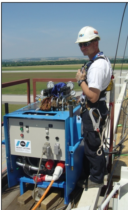
▼ EHP pumps drove the lifting units.
