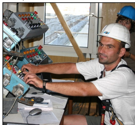
▼ The VSL Bravo control system in operation
