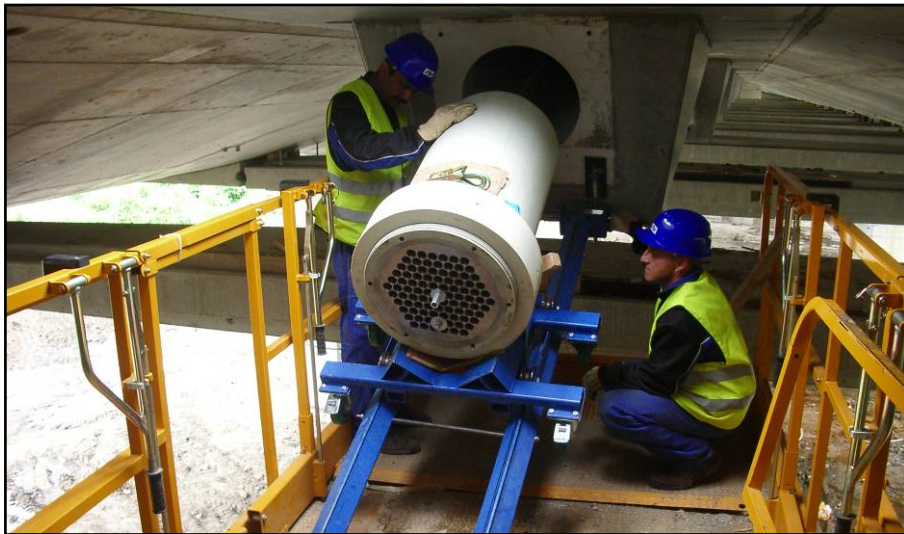
▼ Active anchorage installation
