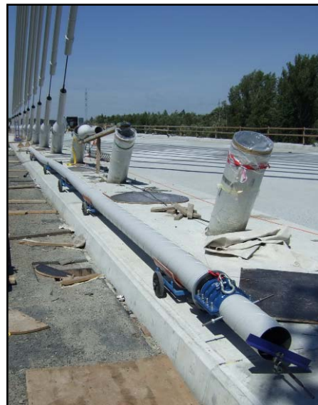
▲ HDPE pipe ready for installation
