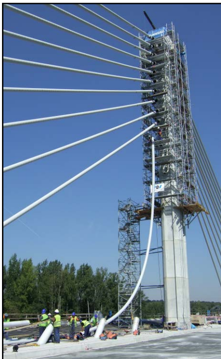
▼ HDPE pipe installation
