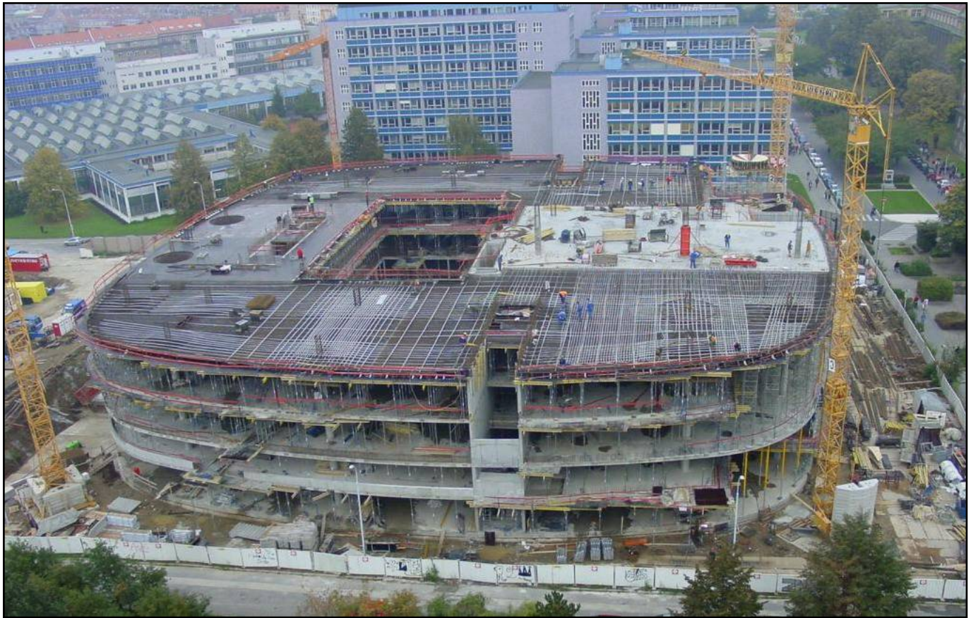
▲ The National Technical Library in the course of construction
