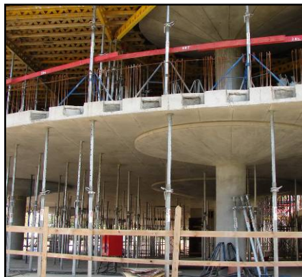
▼ Anchoring pockets after grouting of the tendons
