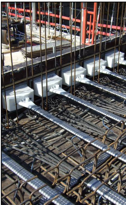
▼ Active and passive anchorages prior to concreting
