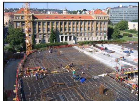
▲ Concreting of sections at various stages of construction
