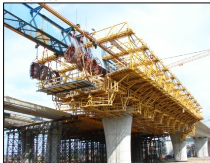
▲ Strand coils suspended on overhead movable scaffolding system.
