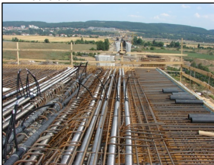
▲ A pier table ready for concreting .
