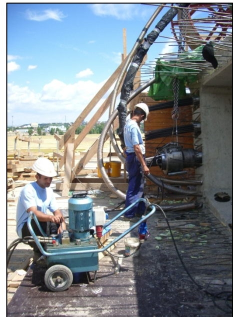
▲ Stressing in a typical construction joint.
