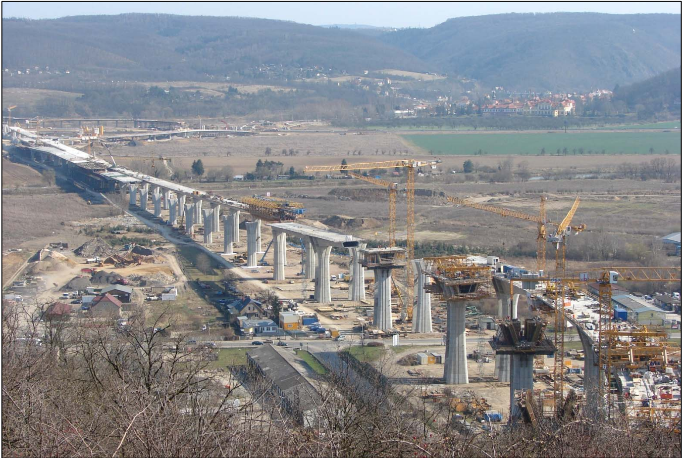
▲ Overall view on the bridging of "514 Lahovice - Slivenec construction, SO 204" section.
