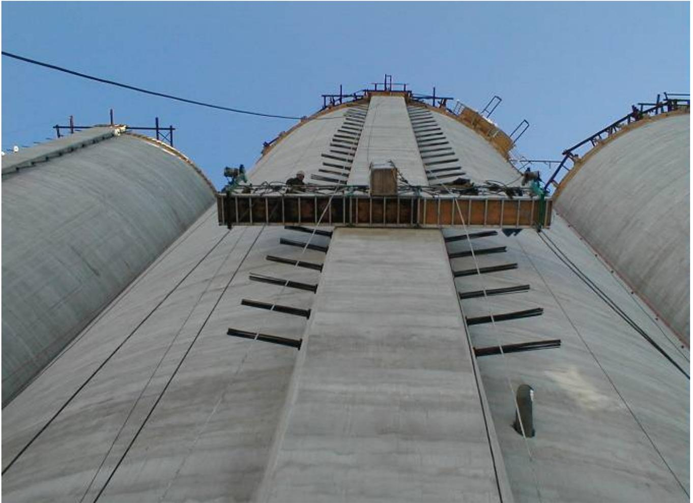
▲ Access to work was achieved using swing stages supported with steel beams placed at the roof of the silos
