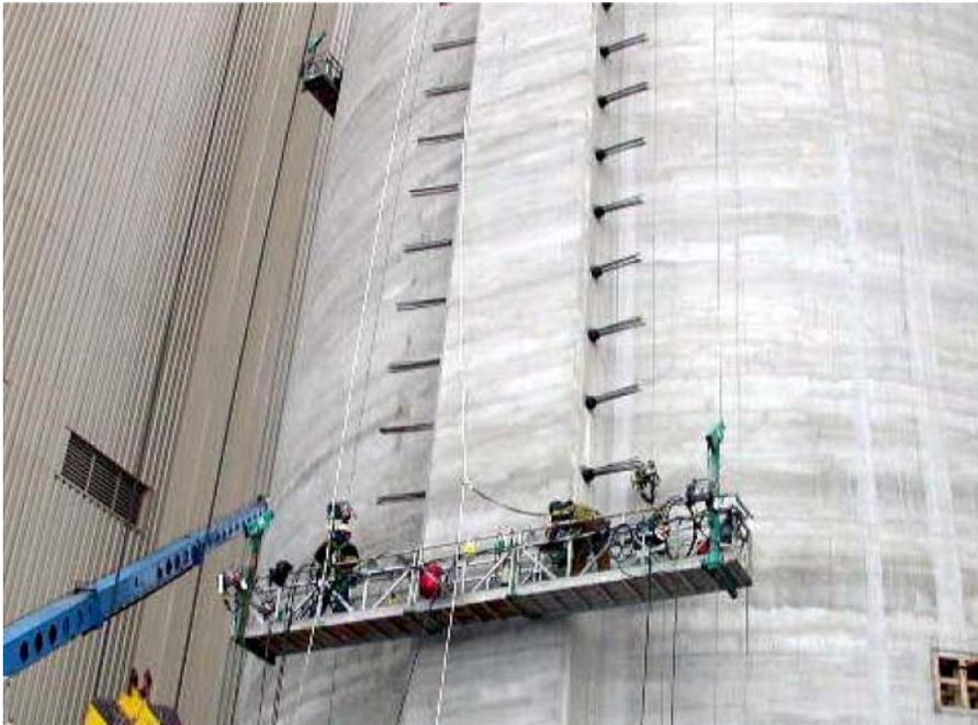
▲ Tendon stressing and grouting was performed after the silos were slipformed
