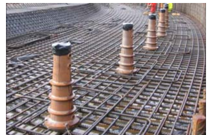
▲ AF Anchorages installed in the slab of the tank
