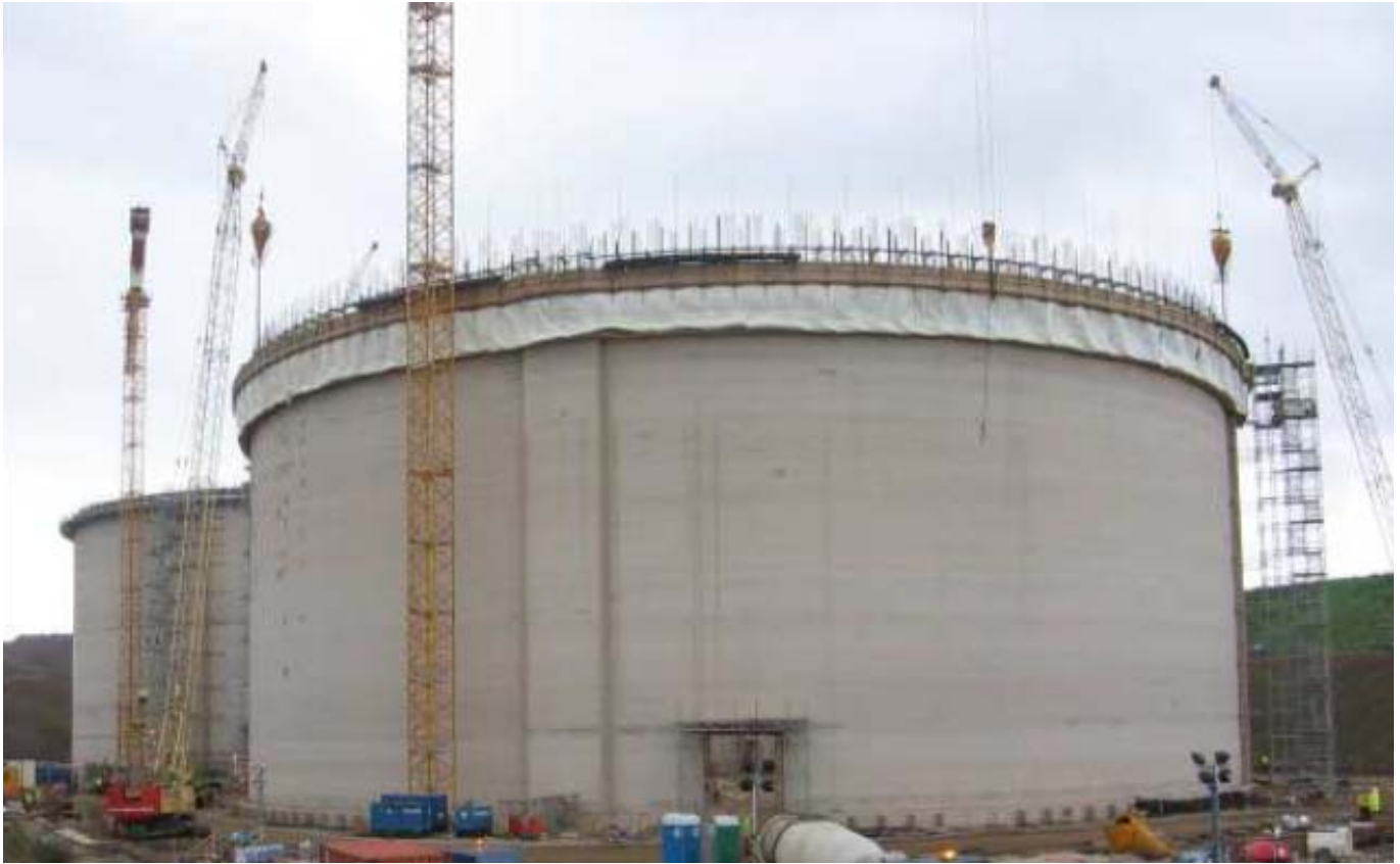
▲ Dragon LNG Tanks during the slip forming
