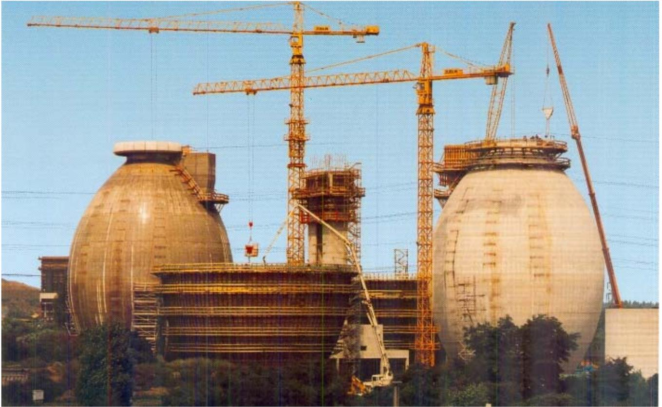
▲ *With a capacity of 15,000 cubic metres, they are the largest tanks of their kind ever constructed*
