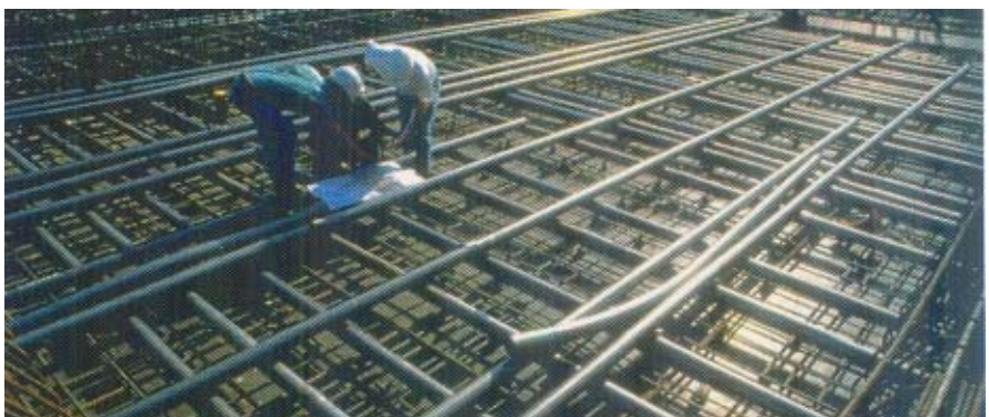
▲ Bottom slab ducts installation
