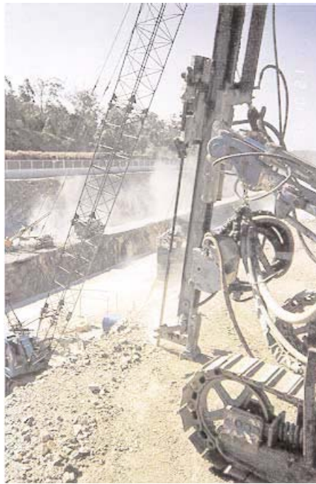
▲ Drilling for chemical anchors
