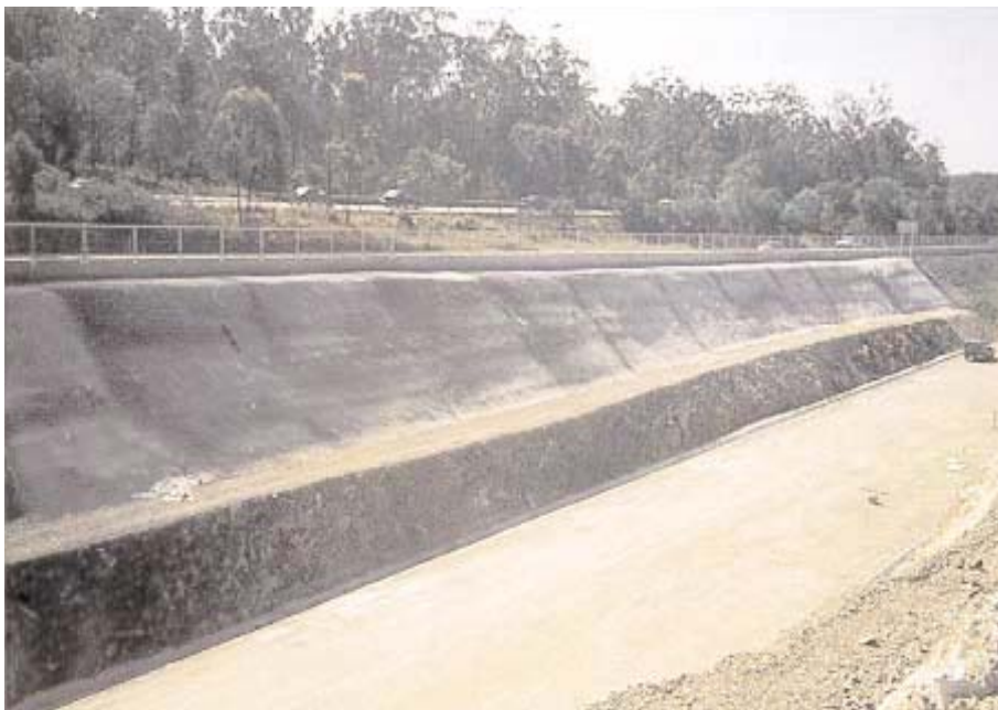
▼ Stabilised cutting with shotcrete facing
