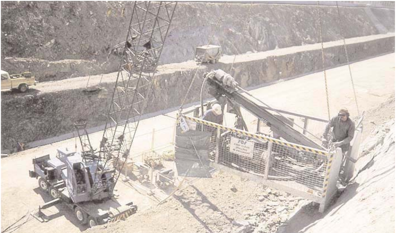
▲ Drilling rig suspended from mobile crane
