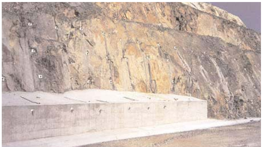
▲ Rock bolted cutting
