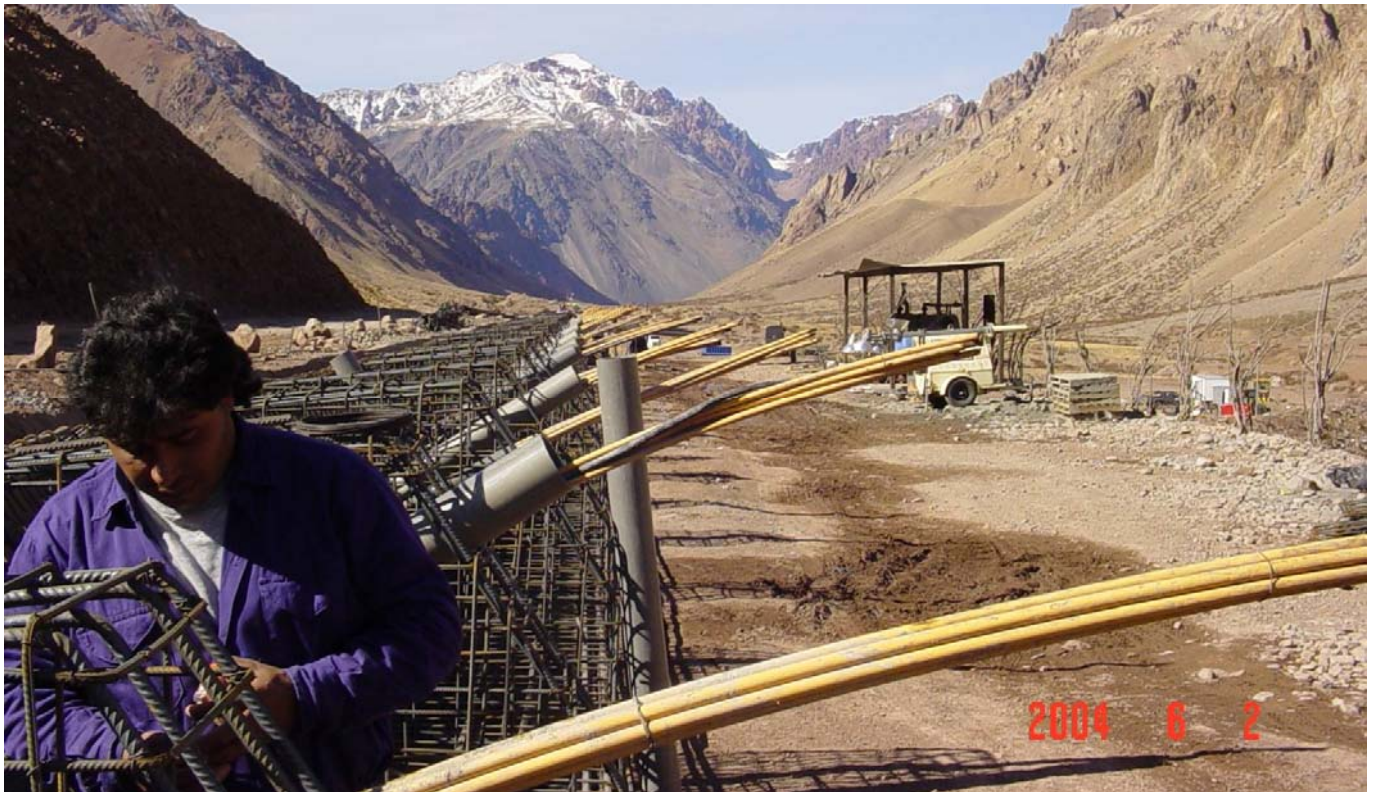
▲ 138 VSL permanent rock anchors as a part of an important road joining Chile and Argentina through the Andes.
