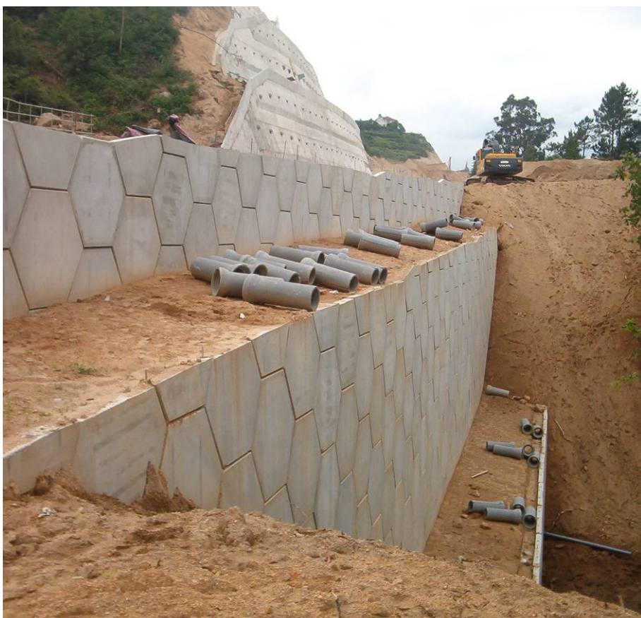
▲ Erection details with various levels of walls
