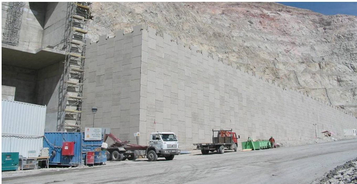
▲ Building a 4,000m 2 36 m high was an amazing goal, the project was built with non-galvanized mesh
