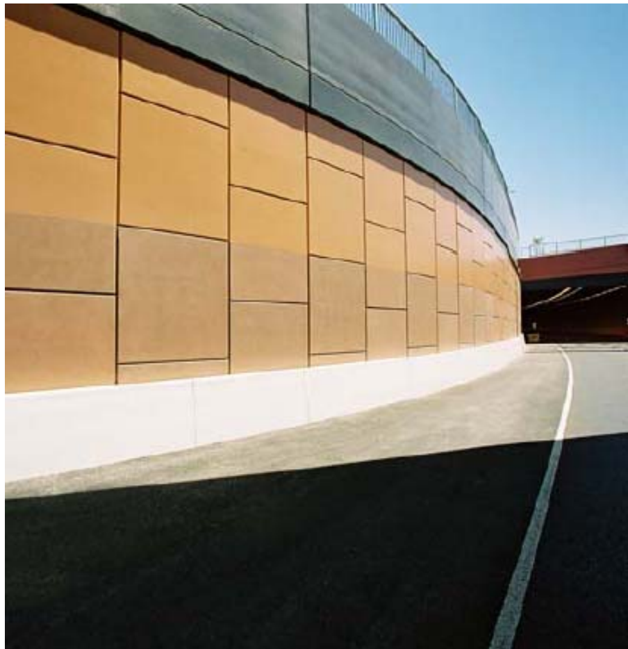
▼ Main Tunnel approach wall for Nundah Bypass
