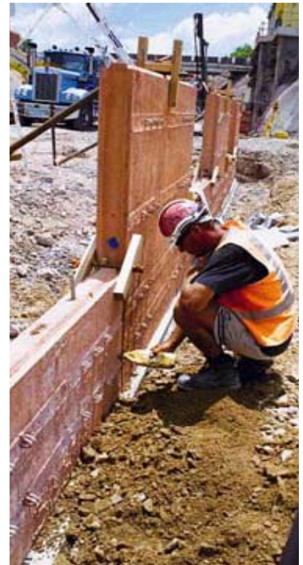
▲ Assembling of panels
