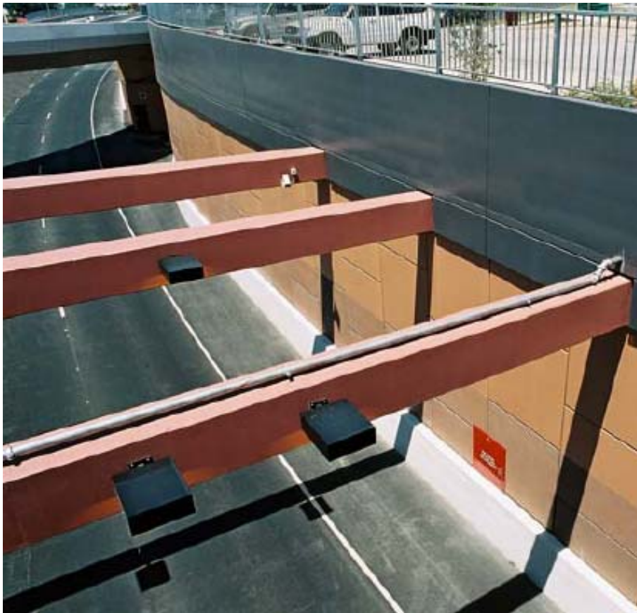
▲ View back to Bridge Structure
