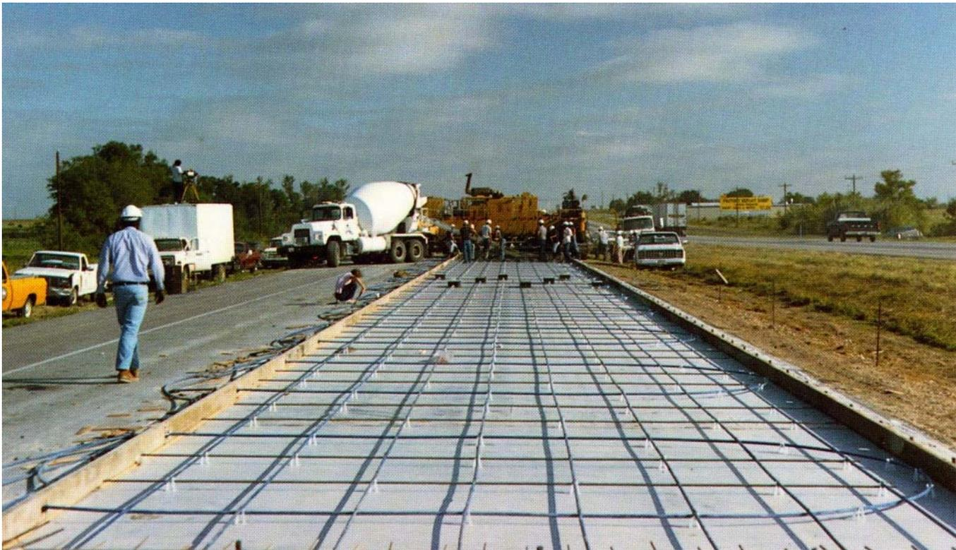
▲ *The prestressed concrete pavement preparation*
