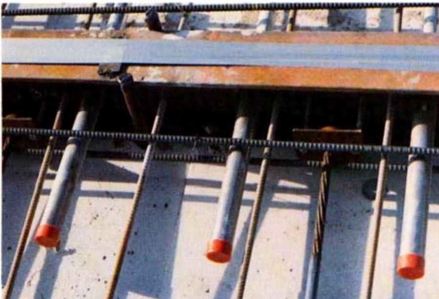
▲ **Stressing Blockouts:** The stressing blockouts were staggered along the center of each slab. Early stage stressing at concrete strength between 1,400 psi and 2,300 psi eliminated surface shrinkage cracks. Final stressing was performed 48 hours after concrete pour.
