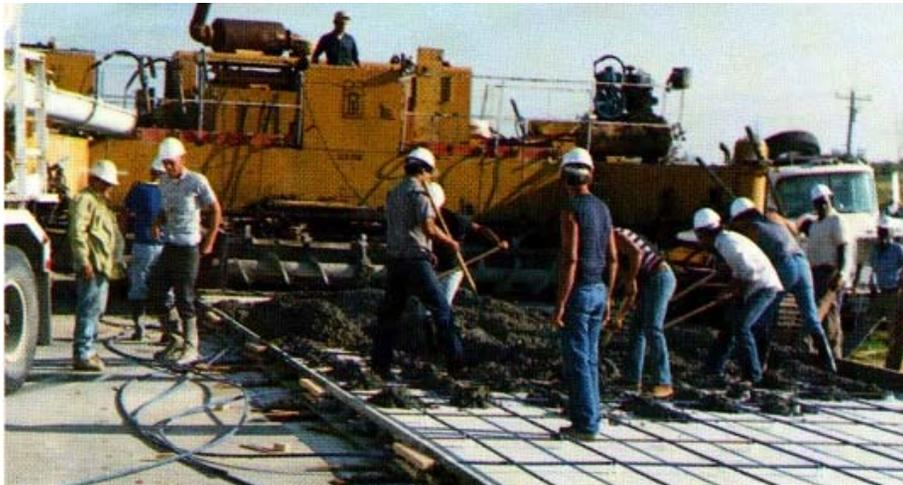
▲ **Concrete Pour:** *A large concrete finishing machine was employed to distribute the concrete evenly, vibrate the pour and finish it.*
