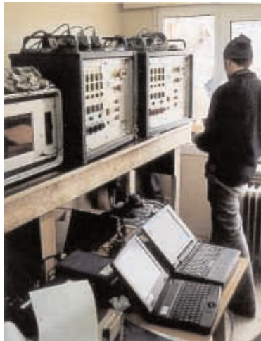
▲ Control room: the nerve centre of the lifting operation
