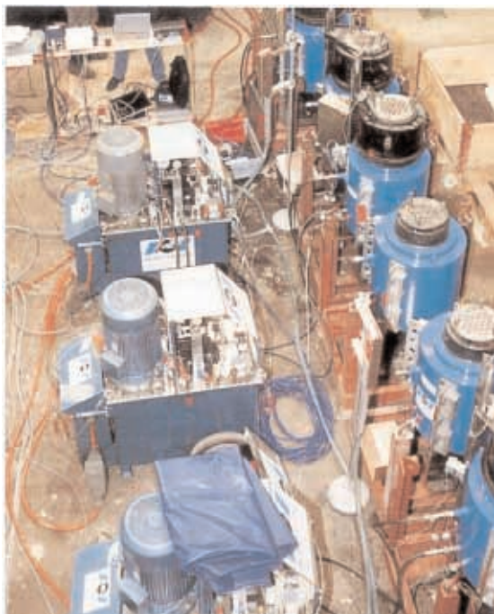
▲ Shop-testing the lifting equipment (partial view)
