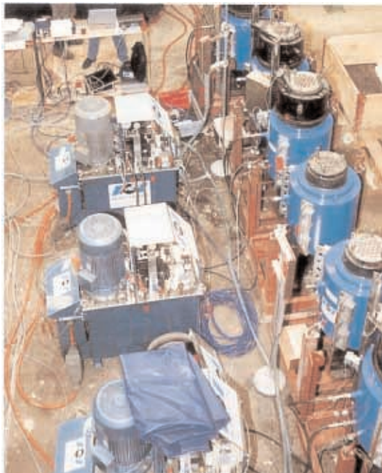
▲ Shop-testing the lifting equipment (partial view)
