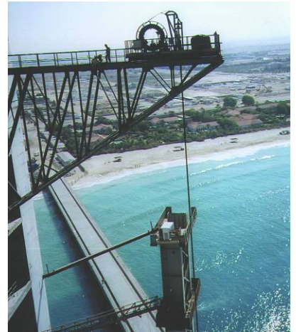
▲ Jacking carriages mounted on cantilever frames
