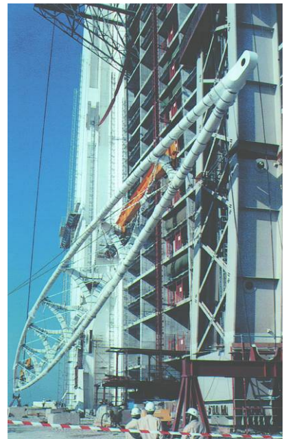
▲ Lifting of prefabricated diagonal truss
