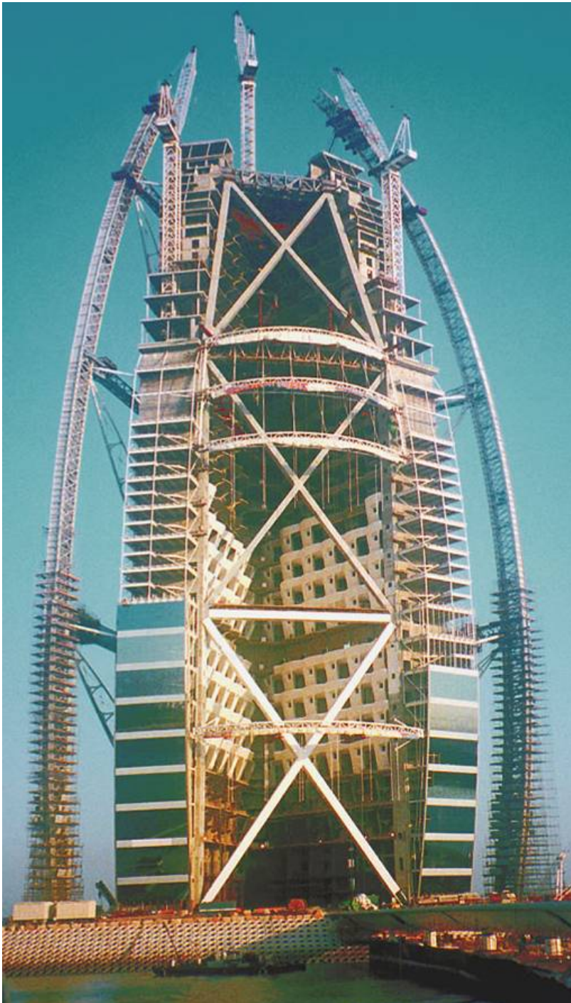
▲ The tower hotel under construction, Chicago beach, Dubai
