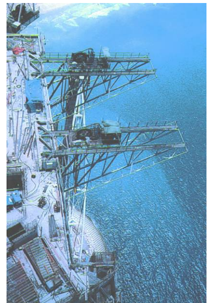
▲ The final stage of truss lifting
