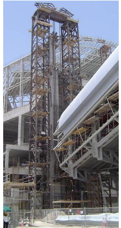
▲ One of the shorter lifting towers. In the background the roof of the lower part of the ski slope, erected in a conventional way.
