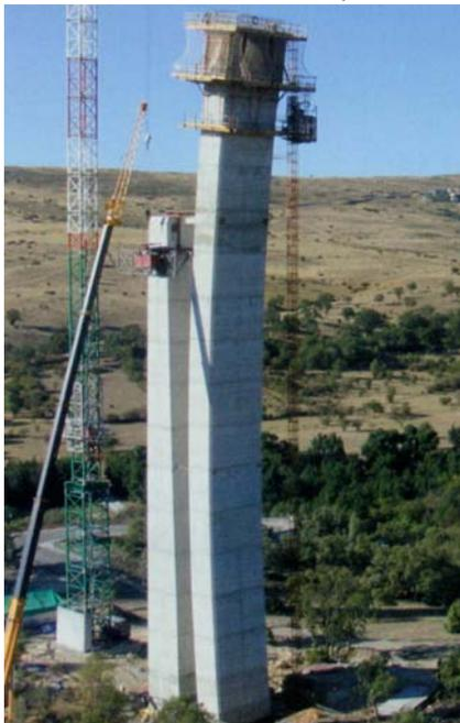
12 strands each that were used in the initial phase to generate a minimum force of 160T in the system and lower the half-arch in a controlled manner.
