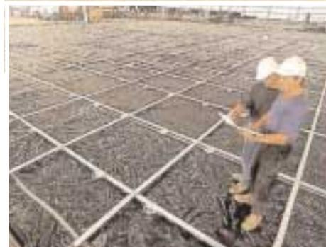
Post-tensioning of 42,000 m<sup>2</sup> of slab on grade greatly reduces jointing in the slab
