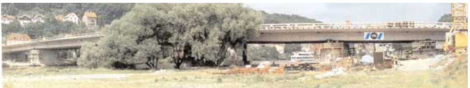
194 m were pushed with bare dry strand over four high points at the piers using VSL's standard pushing equipment, powered by two EHPS 33 pumps. VSL's post-tensioning work was completed within 18 weeks to the full satisfaction of the main contractor Philip Holzmann - Held & Francke Bau AG in the beginning of July 1995. /
