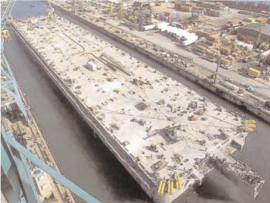
The Nkossa vessel is the largest prestressed concrete barge in the world. The quantities of material used illustrate the gigantic size of this unique floating structure of 25 000 m<sup>3</sup> of concrete built in a record time:
