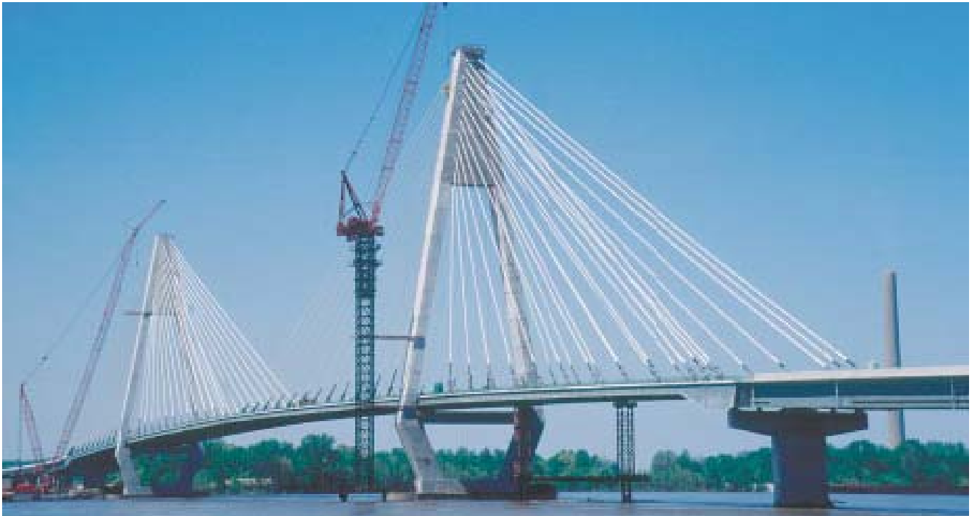
▲ The 4,505 foot-long William Natcher Bridge was the first US bridge to use steel cable anchorages.
