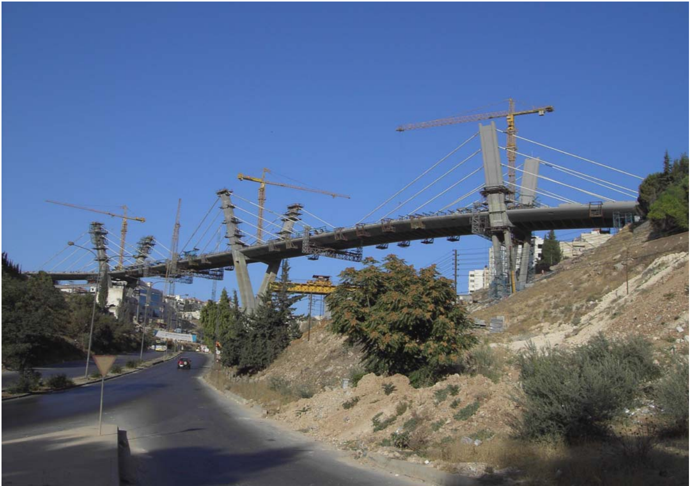
▲ Side tower T1 & middle tower T2
