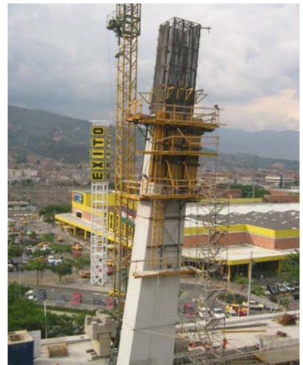
▲ The pylon under construction
