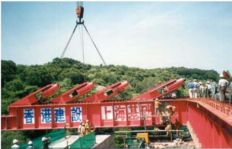
▲ Stay passive and anchorages attached to steel main girder
