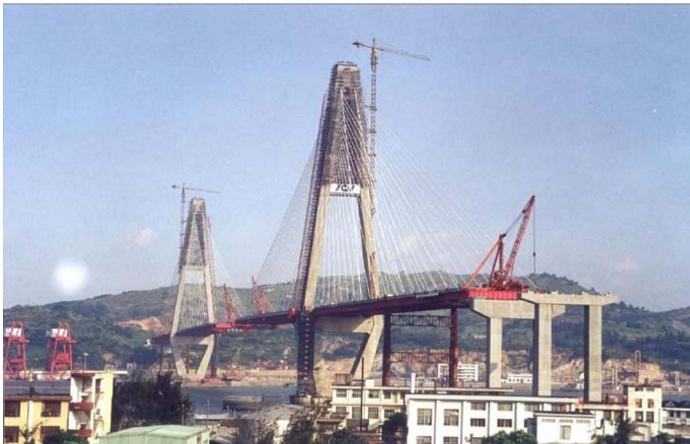
▲ Deck erection and VSL stay cable installation
