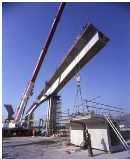
▲ Erection of balance cantilever using cranes
