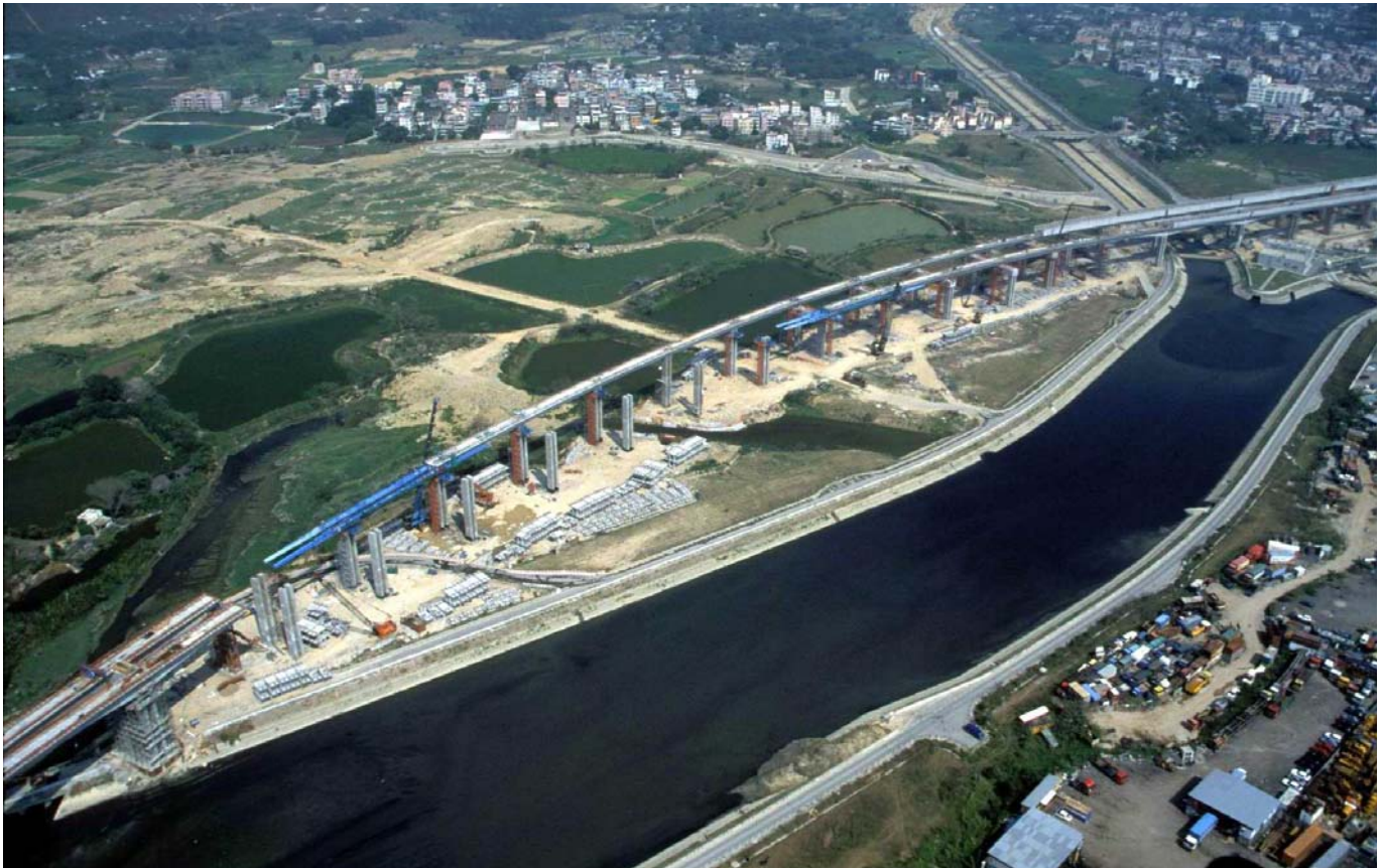
▲ CC201 (Kam Tin) – Two underslung girders working in tandem
