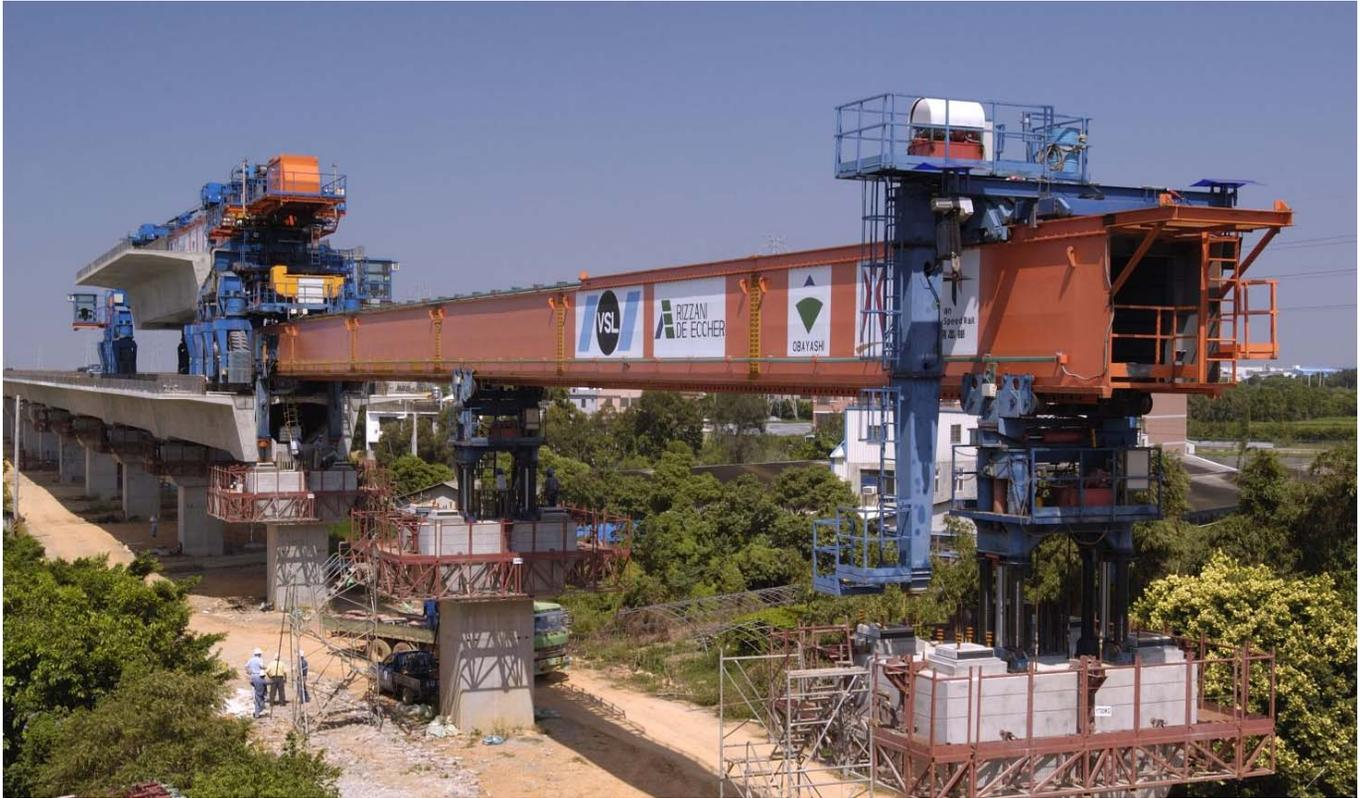
▲ FSPC technique: a speed of erection faster than one bridge span per day.
