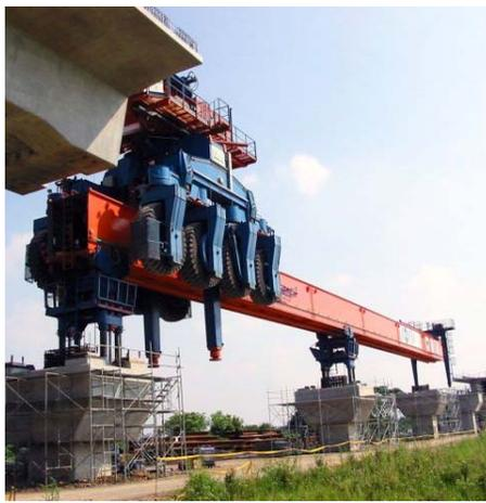
▲ Carrier deployed with 8 tyred bogies supporting an overhead beam
