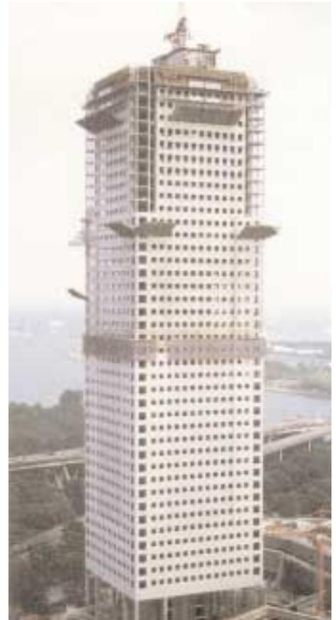
In Singapore, VSL have just completed major post-tensioning and climb-form work for the first tower on the Pontiac Marina (see photo) project and have subsequently been awarded the sub-contract for the second 52 storey tower. On the civil side, VSL are installing the cable stays and post-tensioning for the unique Safti Bridge. /
