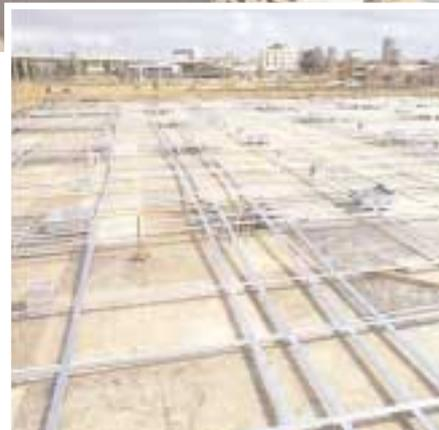
VSL was awarded the design and post-tensioning contract on a 2 way P.T. flat plate alternative slab design, 320 mm thick. All tendons are 5S5 (15.2 mm) slab system.
