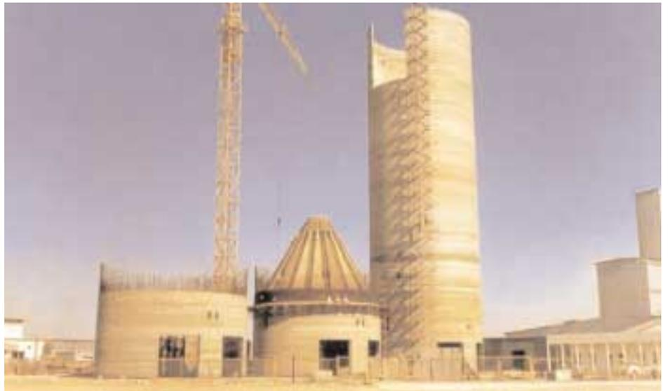
Slipforming in progress on Clinker Silo
