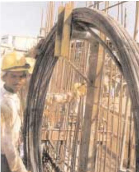
Reeled monostrands being installed during slipforming
