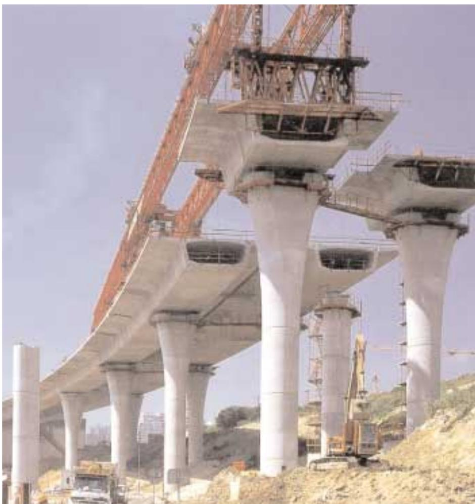
The 1.2 km long Rambler Channel bridge will link Tsing Yi Island's Chung Ching Tunnel with the Kwai Chung Viaduct on the Kowloon mainland. Dual 3-lane expressways are constructed by an overhead launching gantry, placing precast segments using the balanced cantilever technique. Construction began in 1993 and is due for completion by 1996.
