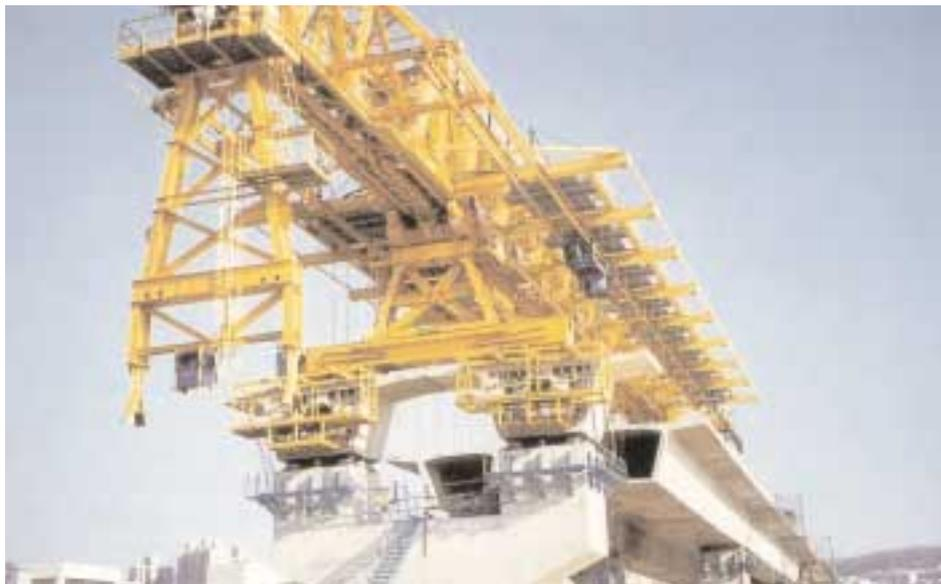
Span-by-span erection using one overhead truss covering two box lines simultaneously
