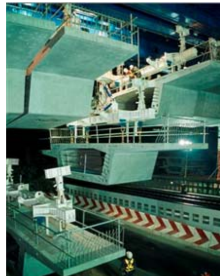
▼ Precast segments suspended above rail tracks
