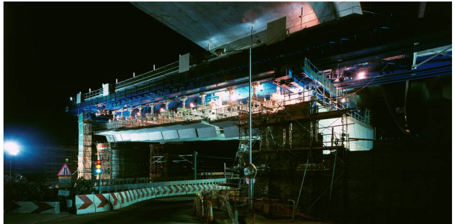
▲ Segments were delivered from below, adjacent to the railway track
