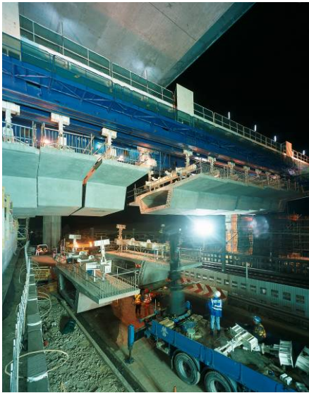
▲ Segments were delivered from below, adjacent to the railway track
