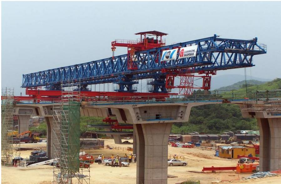
▼ The girders were capable of achieving a 4-shift cycle per span
