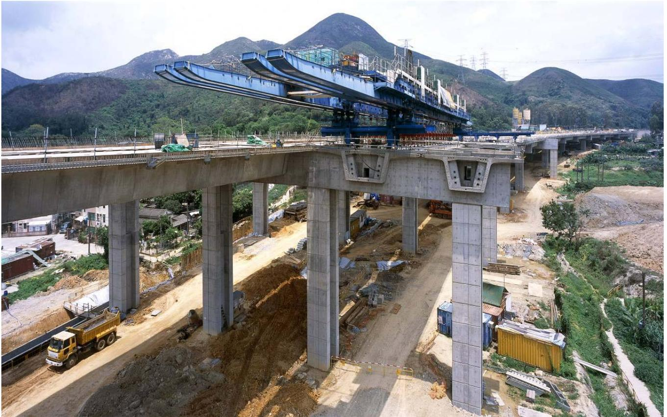
▲ Launching gantry on twin decks of Deep Bay Link viaduct
