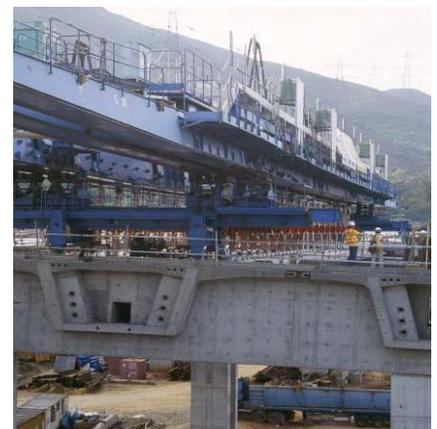
▲ The chords of the launching gantry are 85m long, twice a span length
