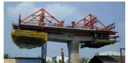
▲ VSL form traveller crossing antique houses.
