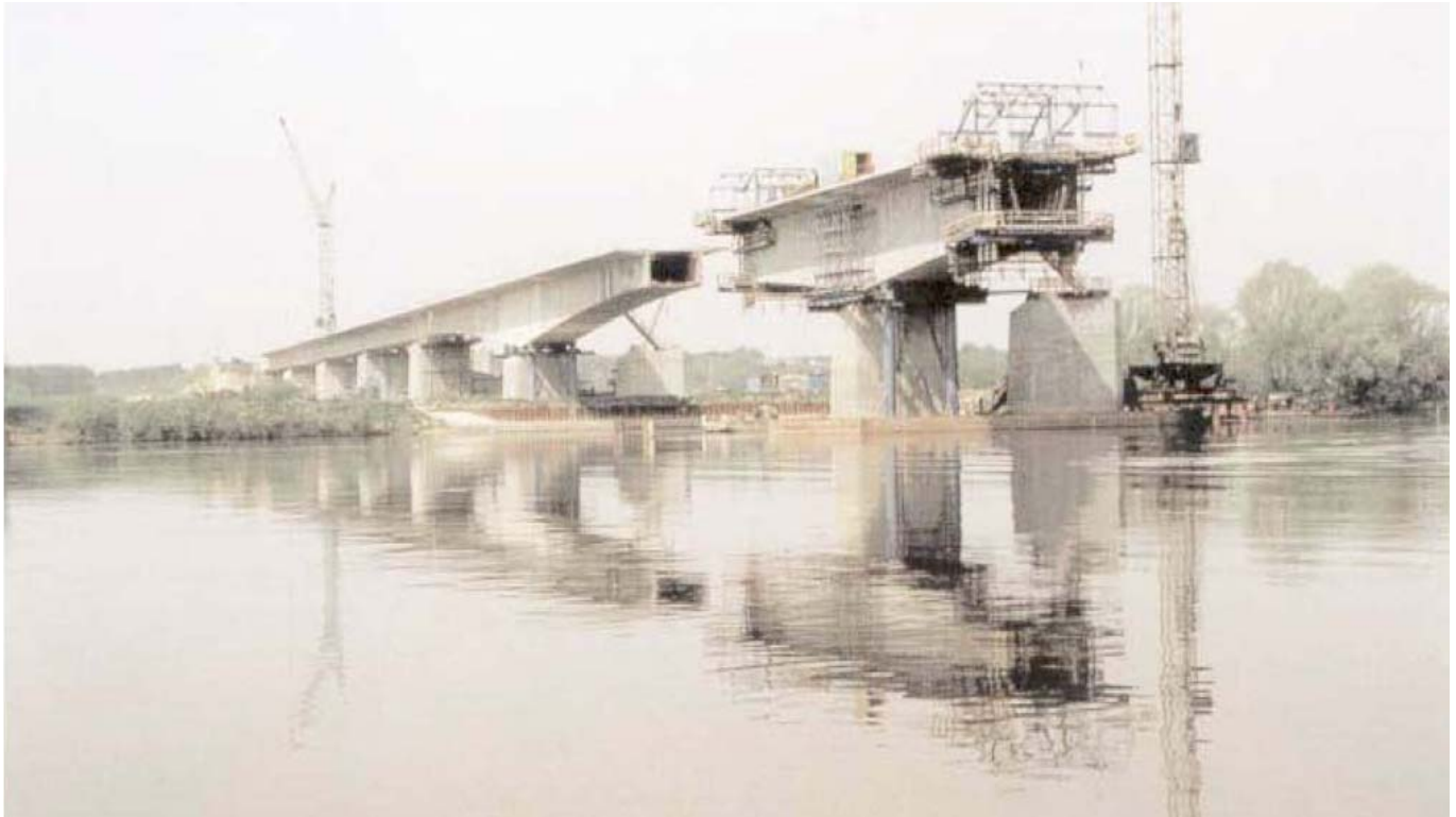
▲ General view of the bridge
