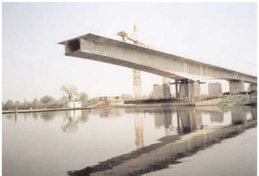
▲ The balanced cantilever section spanning the Vistula river
