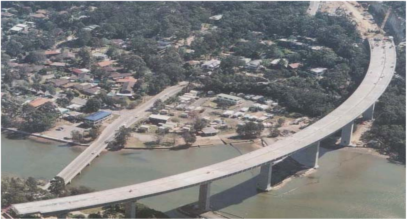
▲ Bridge in final position
