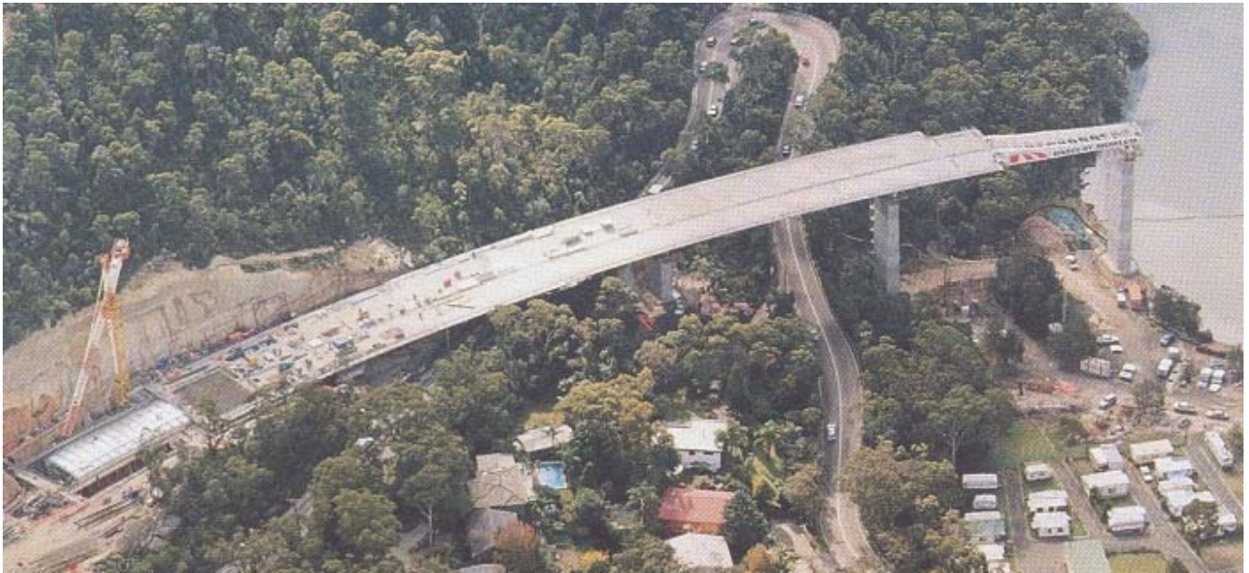
▼ Bridge during launching
