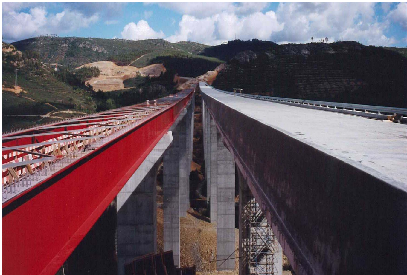
▲ Perdigão Viaduct with 600 m length
