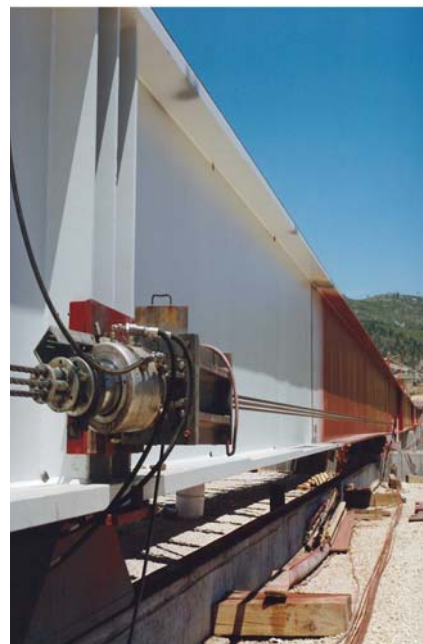
▲ SLU jack connected to the steel girder
