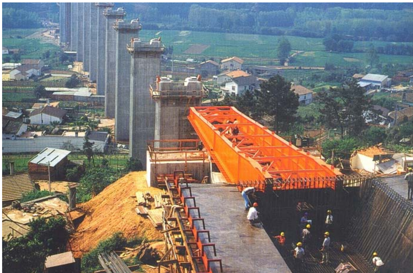
▲ The deck is 856-m long and includes 14 standard 51.5-m long spans
