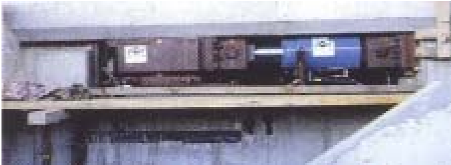
▼ VSL Jacking (lifting and pushing) system under operation
