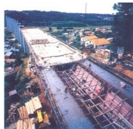
▲ The deck is post-tensioned longitudinally
