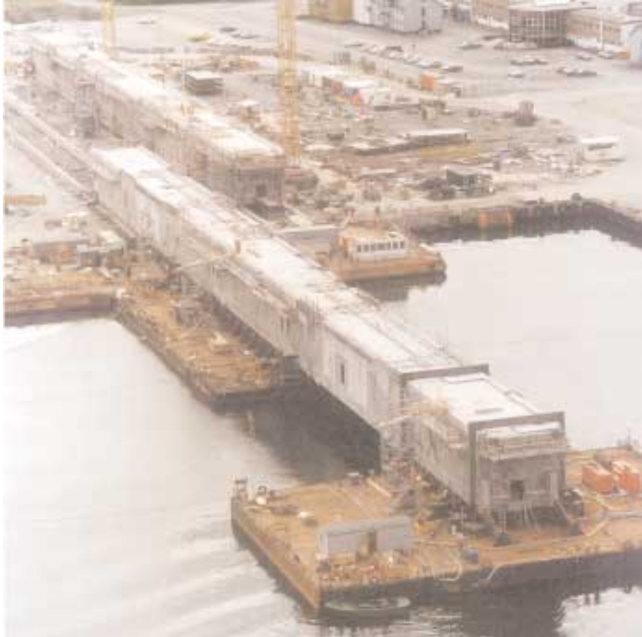
The first module support beam during launching
