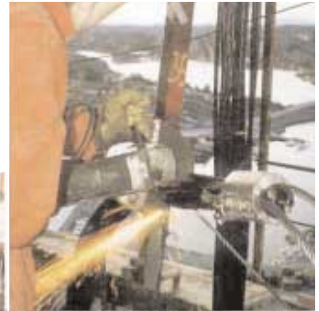
Installing vertical tendons in a column
