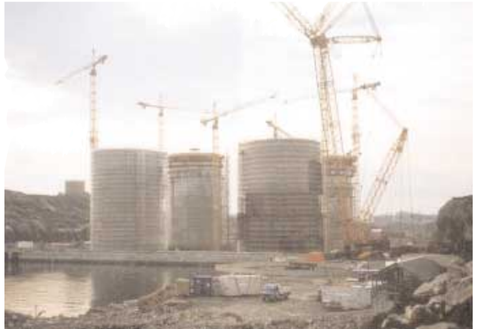
Slipforming of the columns almost complete
